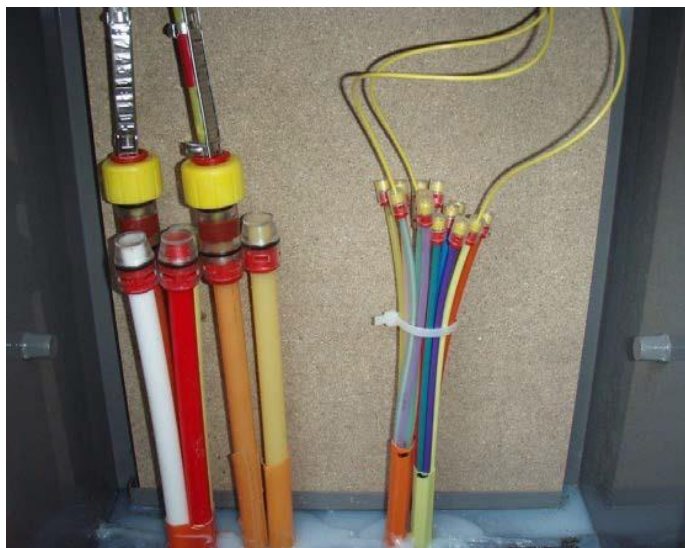
Example of correct sealing of duct
