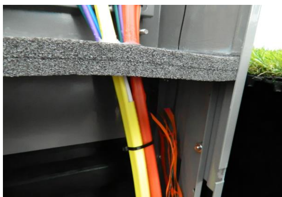
Example of correctly slotted casing
