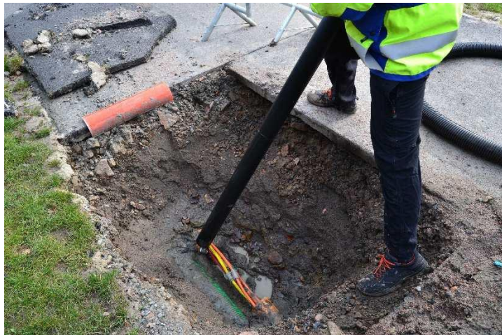
Example of suction excavation by existing cables
