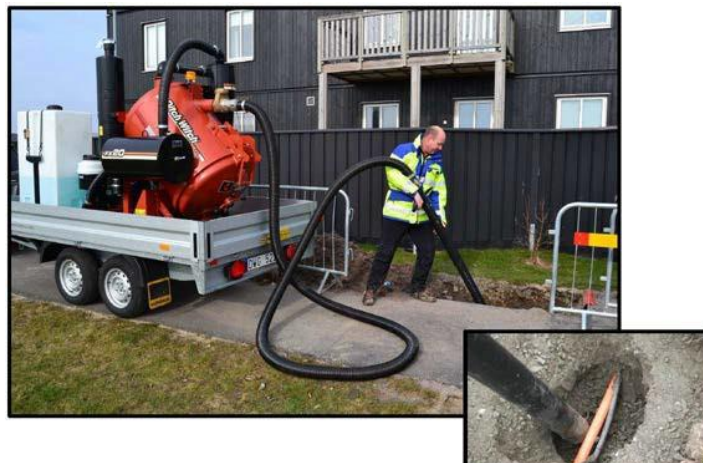
Examples of suction excavation
