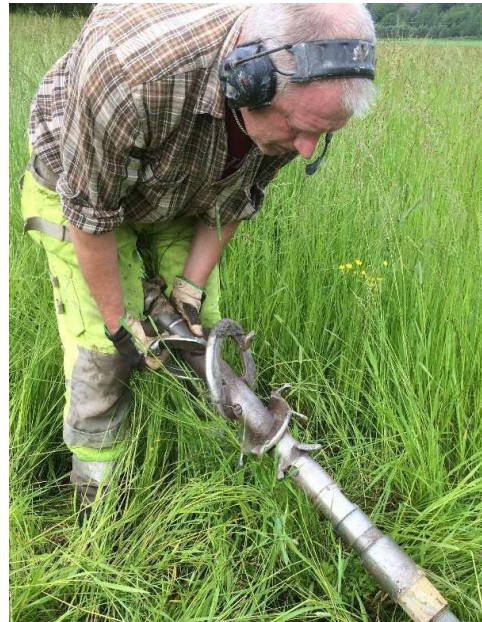
Hole opener installed on pilot rod
