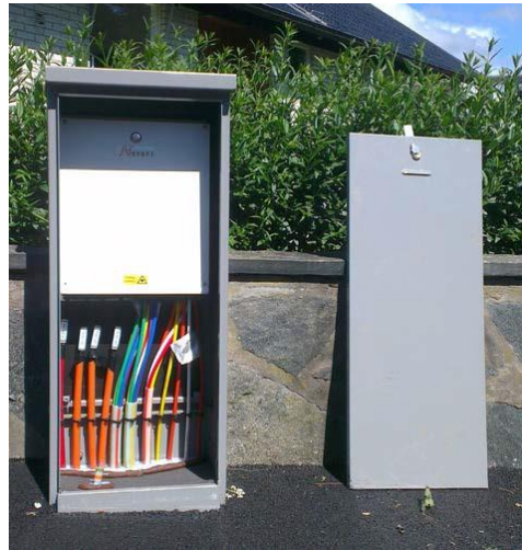
Example of outdoor splice cabinet with splicing unit
