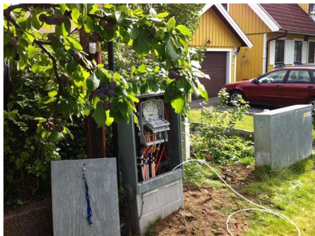
Example of outdoor splice cabinet for outdoor use with splicing unit
