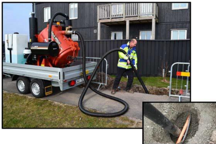
Examples of suction excavation
