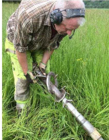
Hole opener installed on pilot rod
