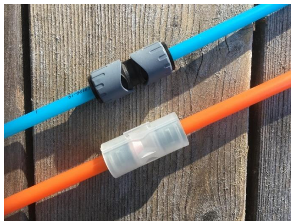
Examples of splicing of microducts
