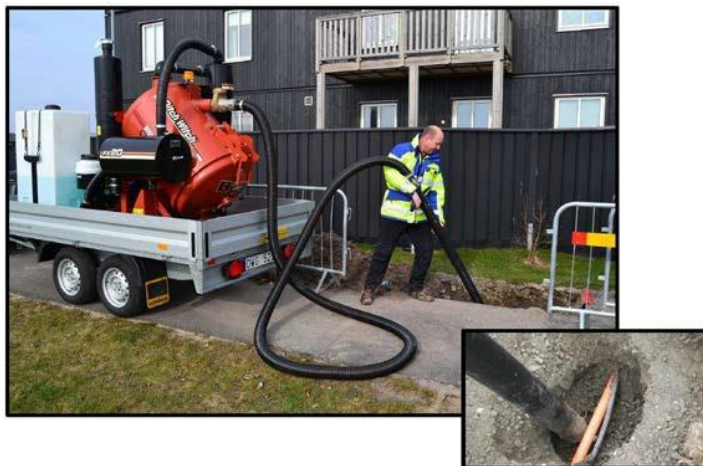
Examples of suction excavation
