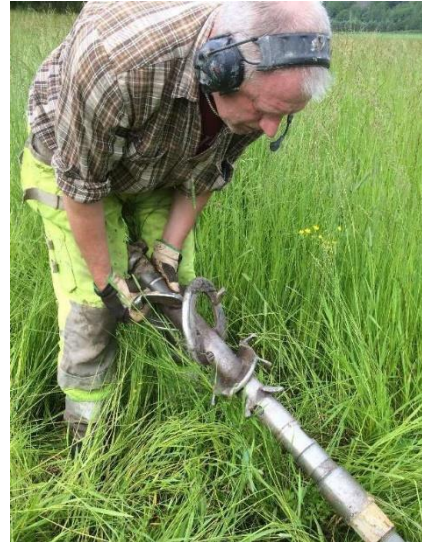
Hope opener installed on pilot rod
