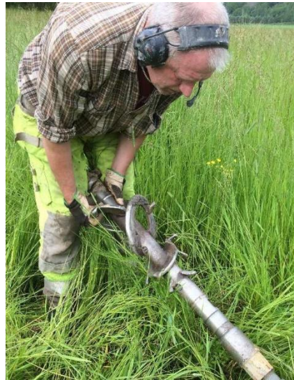
Hole opener installed on pilot rod
