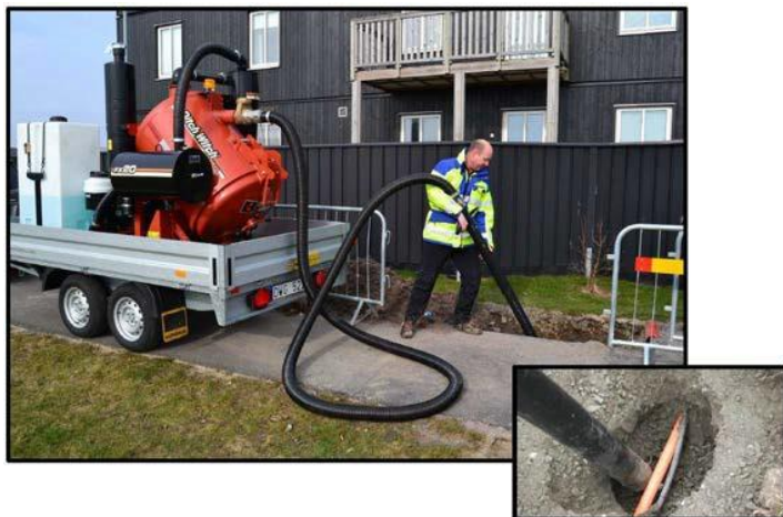
Examples of suction excavation
